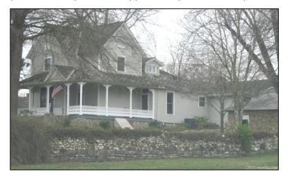
balustrade is also scroll-sawn, and there are decorative vents in the gable ends. The large brick chimney on the south side of the house has corbelled shoulders. The house is supported by brick piers, which have been infilled with field stone. Over the years, several additions have been made to the rear of the house.
